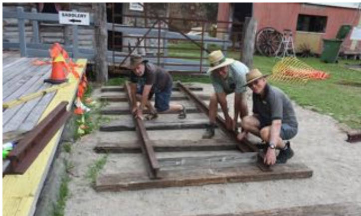
Laying the track.
