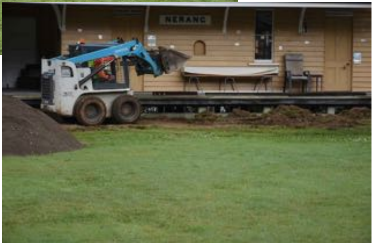
Levelling the site and laying base.
